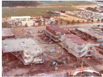
→ First O&G engineering and construction work - a set of living quarters
