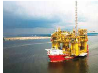
→ Gumusut-Kakap Semi-Submersible Floating Production System (FPS)
