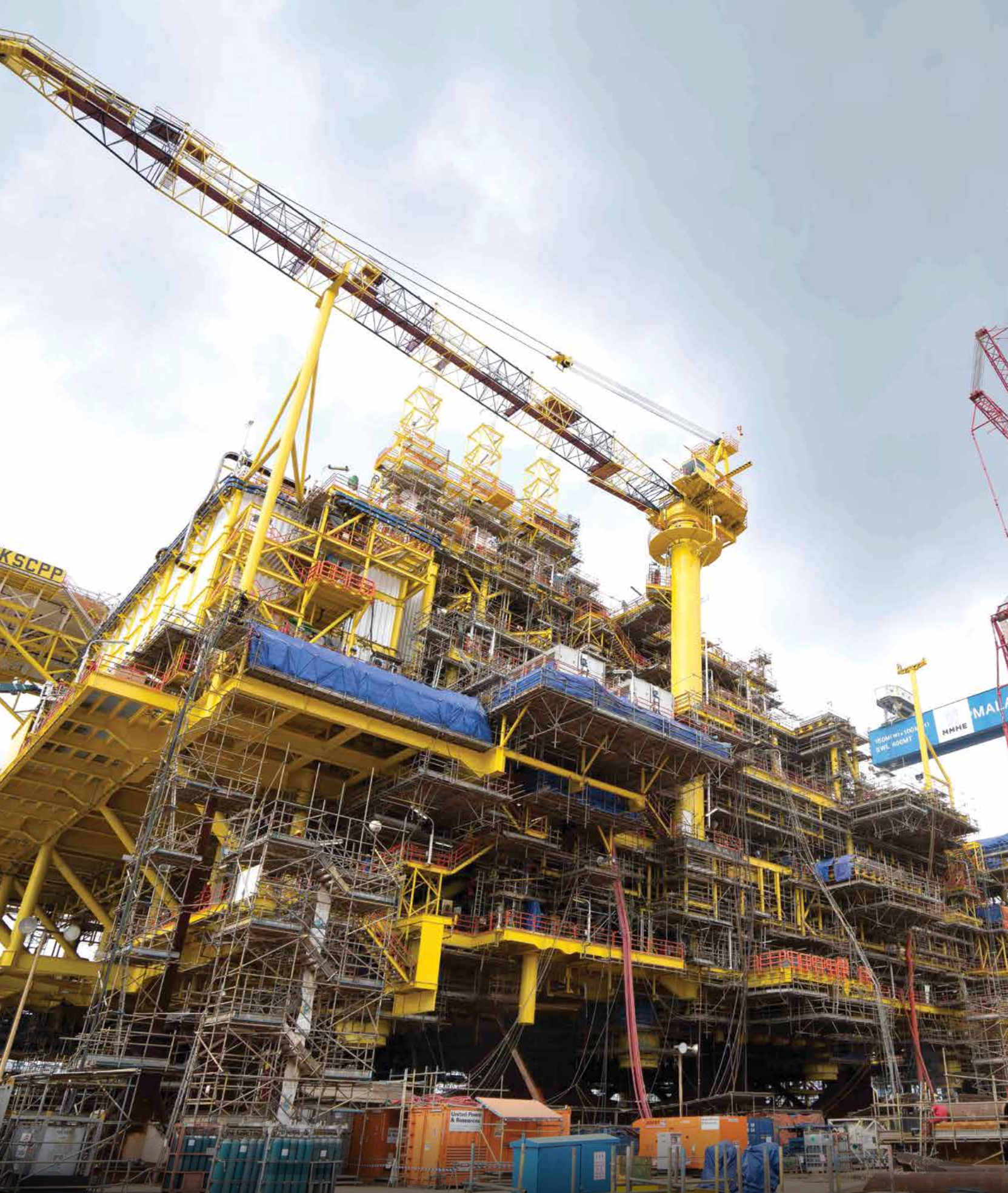
→ The construction of Kasawari Gas Development Project's central processing platform (CPP).
